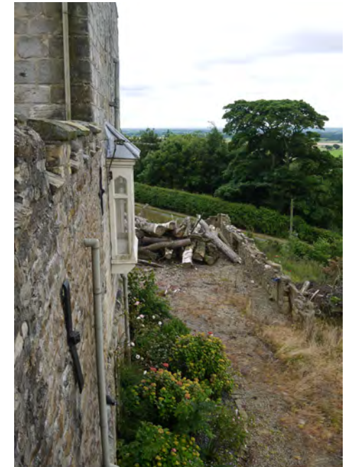
Looking south towards position of former building - lower portions of the south and south-west walls are fossilised in the retaining wall.
