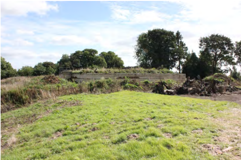
Redundant reservoir with concrete structure stripped of overburden
