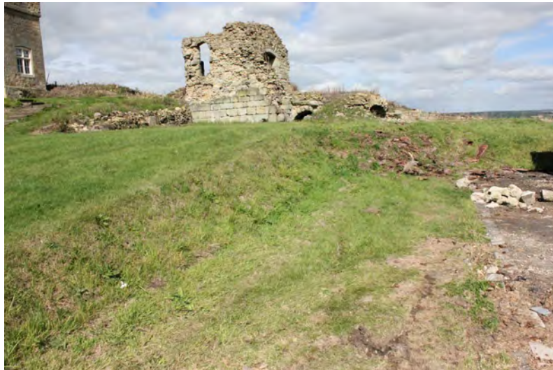
Western edge of levelled tennis court with New Tower behind
