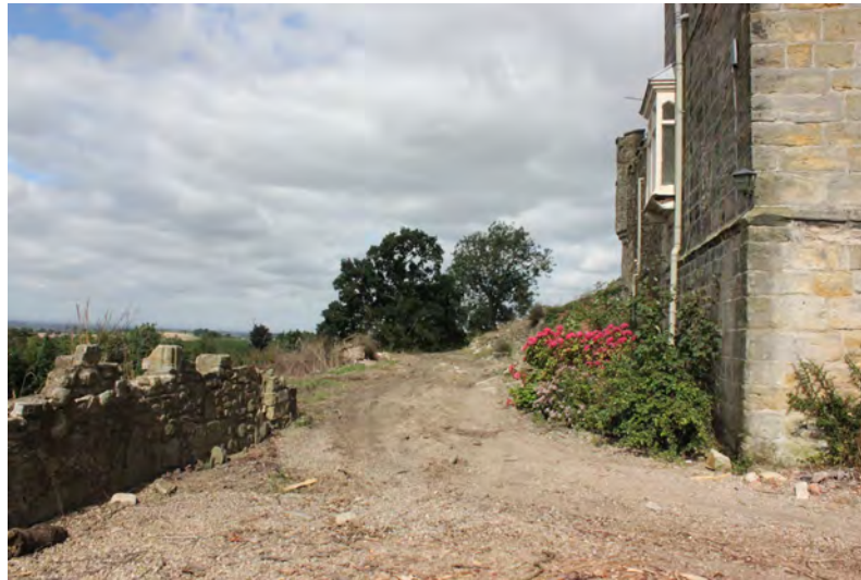
Terrace below western elevation and remains of demolished building to the left
