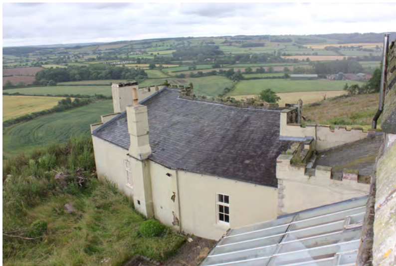
Western elevation of the Victorian extension
