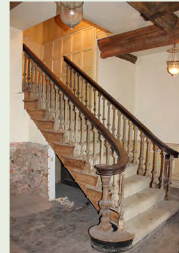
Stair - note the termination of the handrail on the first landing
