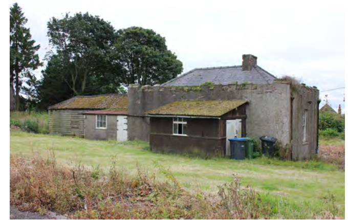
Garage and stables, northern elevation
