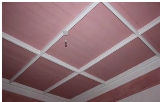
Typical ceiling. Second floor
