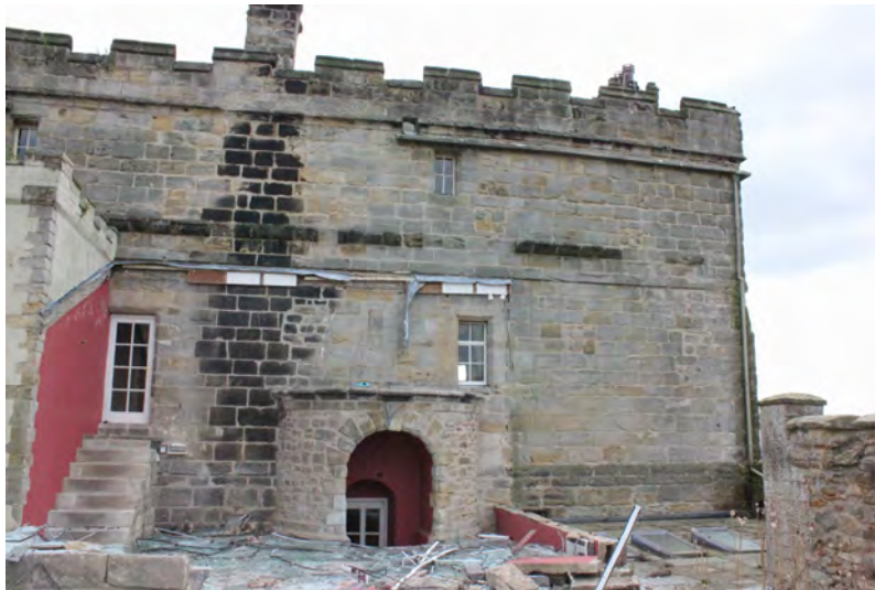
Northern elevation following removal of modern conservatory in 2016
