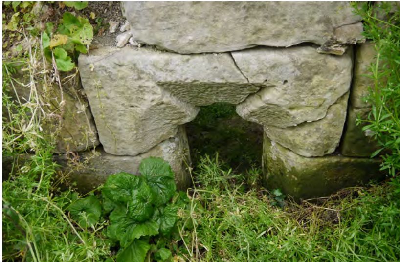
Shouldered window to basement (see page 46 for an historic depiction of this window)
