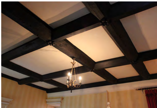
Sitting room ceiling
