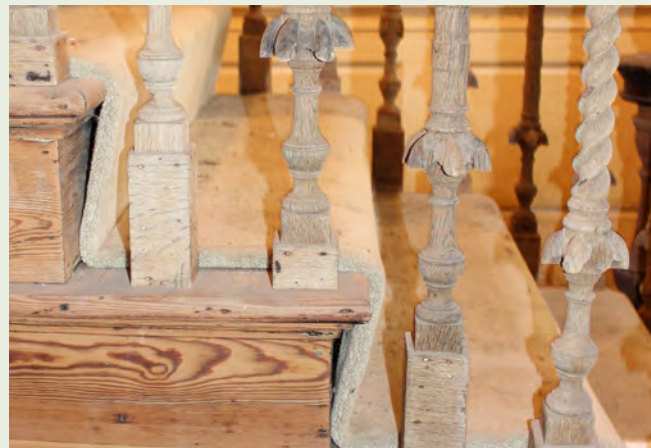
Detail of base of balusters and plain tread ends
