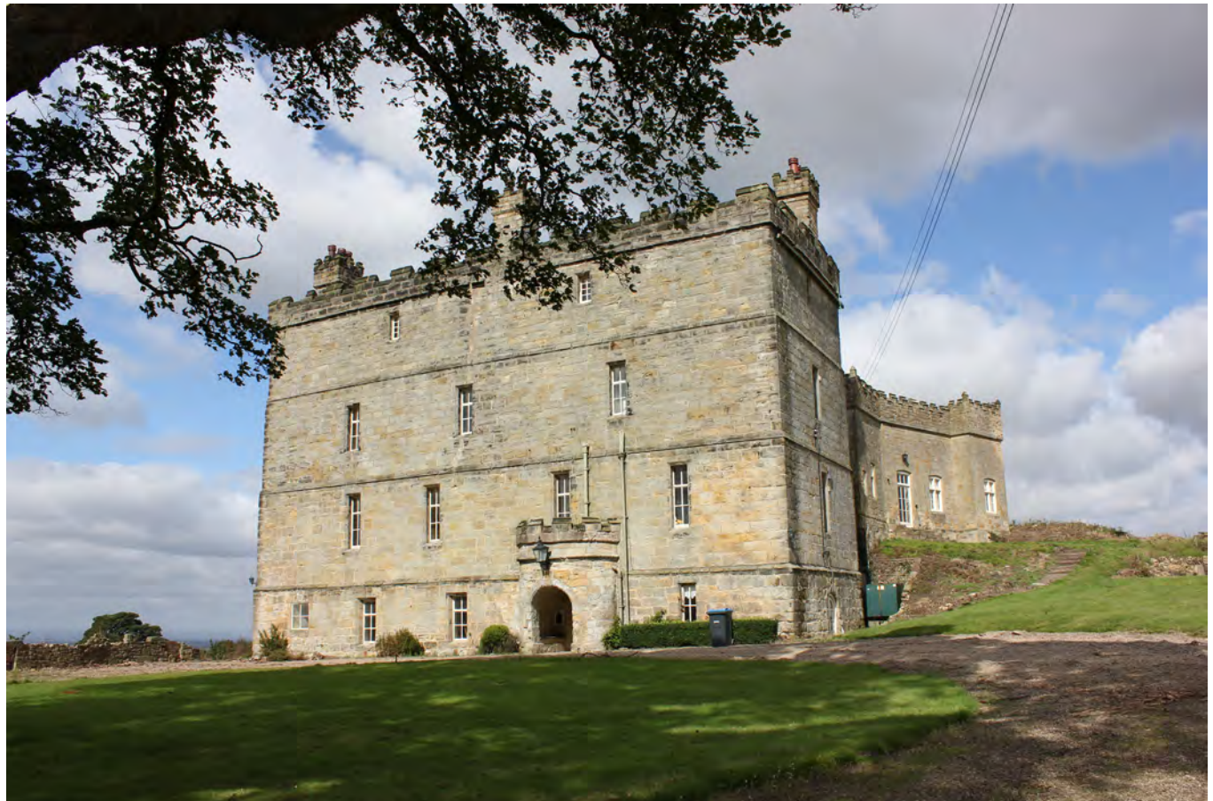
Southern elevation - Victorian extension to the right
