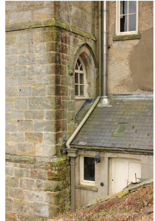
Medieval first floor entrance historically accessed via external stairs (now a window above nineteenth century porch)
