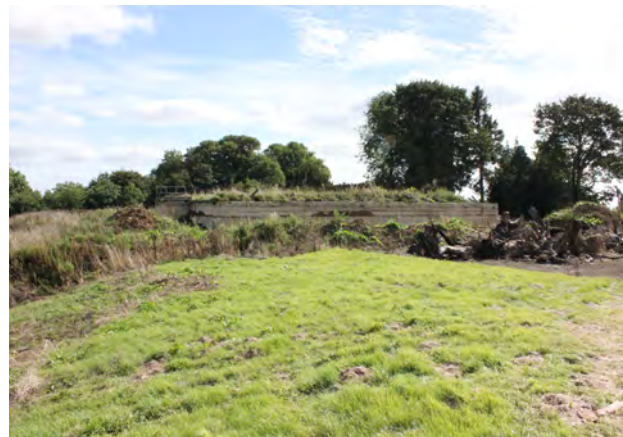
Redundant reservoir with former tennis court to the right. Looking east.
